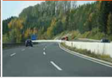
Road stabilised with Geotextiles
